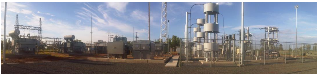
Figure 2: Ergon's St. George Hybrid D-VAR ® STATCOM Installation
